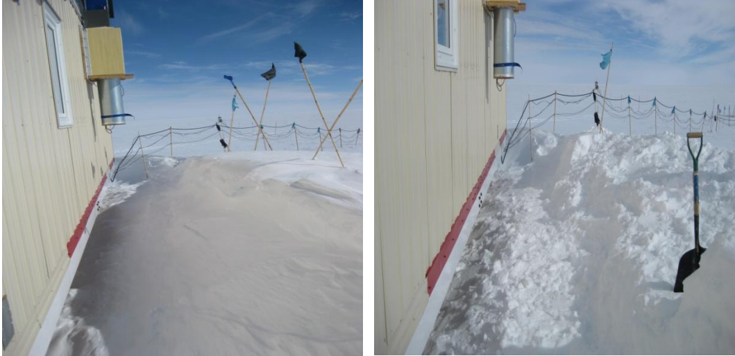
South MSF drift maintenance. -CVH
