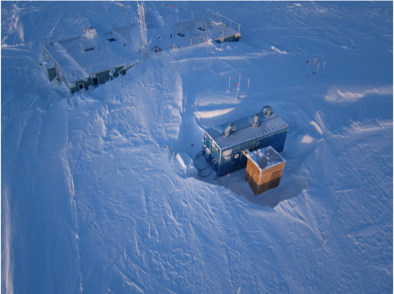
Snow drifts rise around the Green House and microturbine buildings. SWD.
