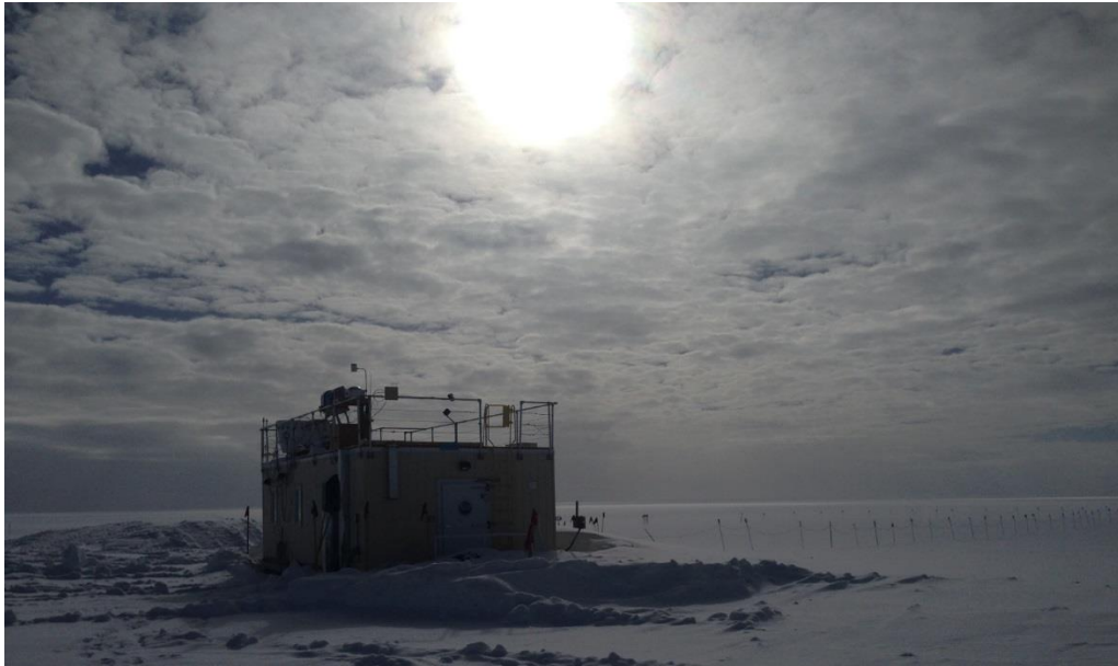
The new MSF pad behind the building has slowly grown over the last few weeks, and later in the coming week the building will be relocated to sit 2 meters above grade. -HJ
