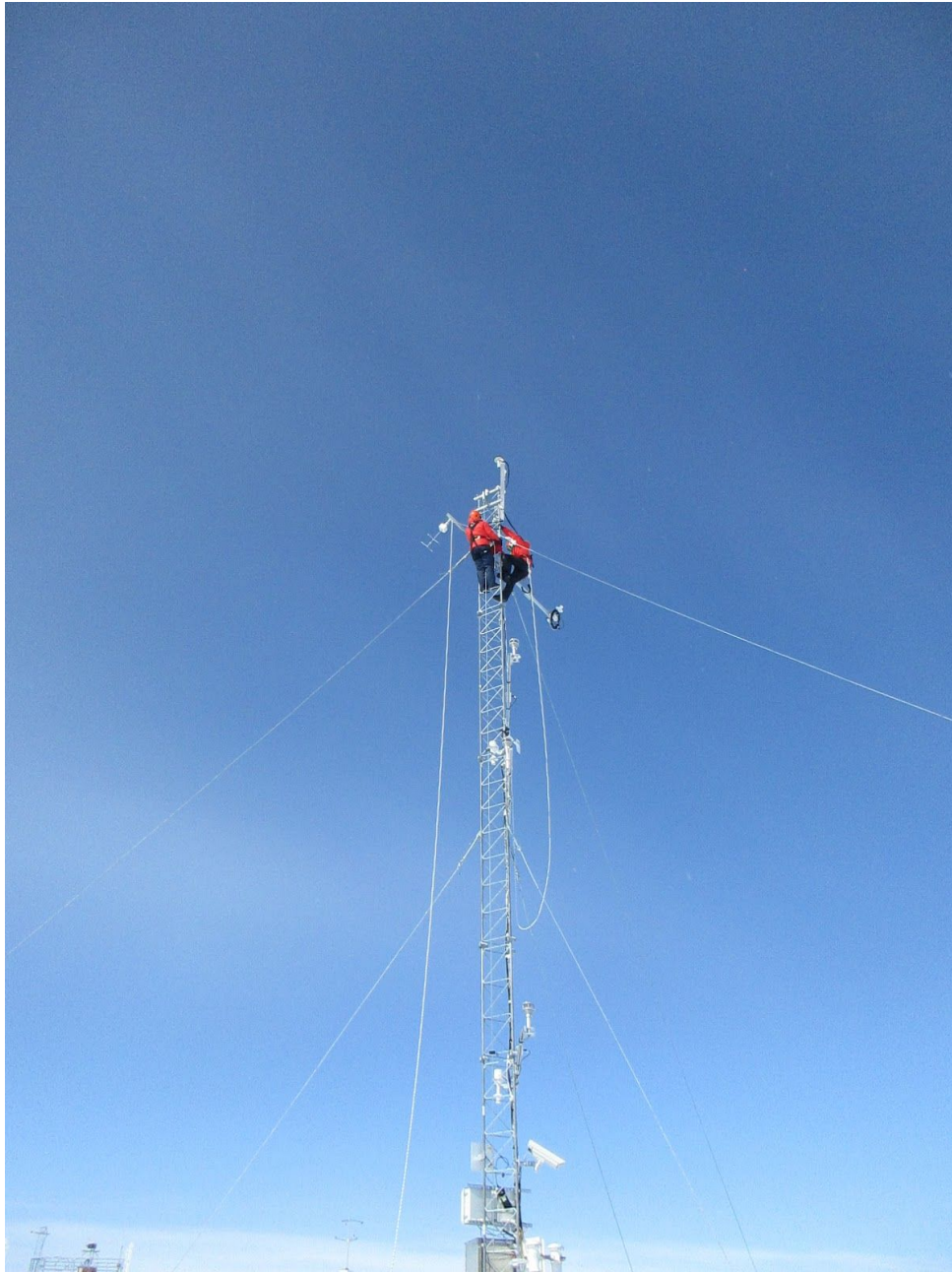
Heather Guy and Bethany Wyld installing an Instrument Boom on the TAWO Met tower.
