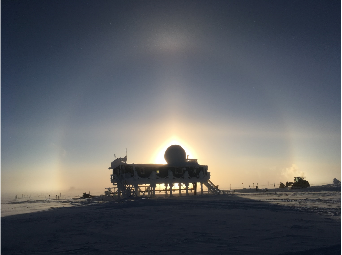
Faint solar optics on 3-4 provide a nice backdrop for digging out the freezer trench and thawing the BH sewer outfall.
