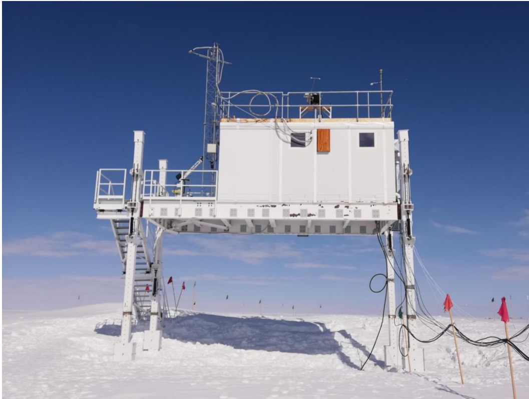
TAWO building after 8.5ft lift. Note INP inlet is now unobstructed (top right).
