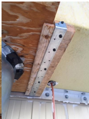
Left to Right: The crack “before”; the crack “after”; a happy PAERI fan hood (attachment reinforced too).
