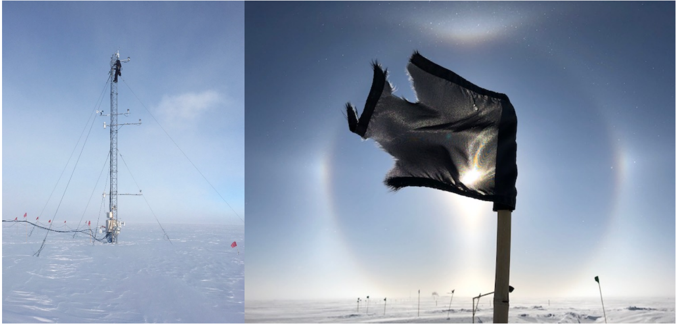
Left: Nate continues inspection of fluxtower systems. Photo Mara Menahan. Right: Solar optics on 2020-03-30. Photo Nate Bowker
