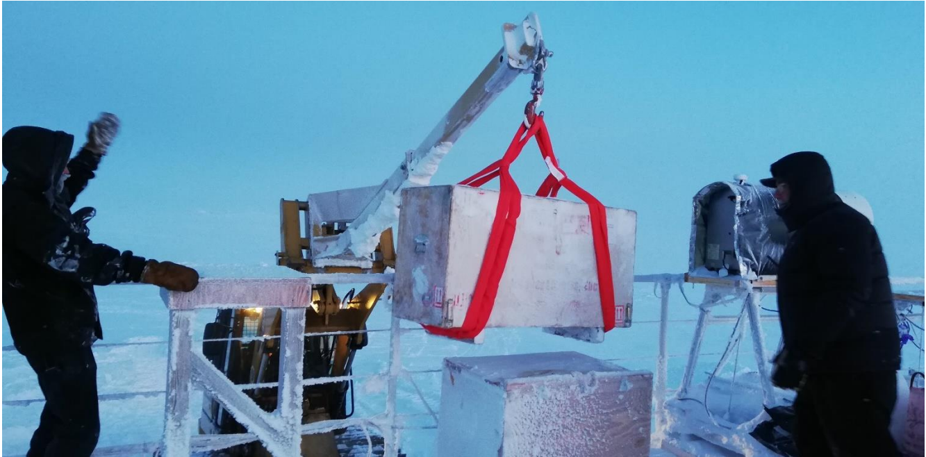
Removing the HATPro from the MSF roof for troubleshooting, 2020-11-20.
