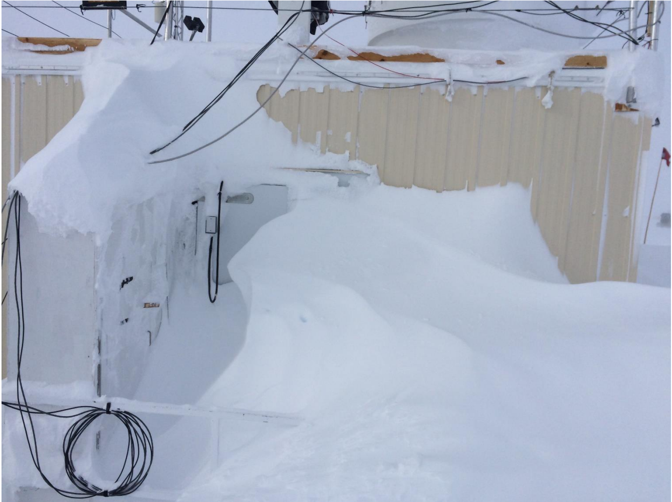
The backdoor of the MSF following the most recent wind event.
